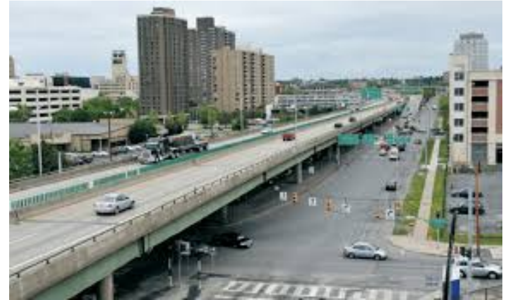
I-81 Viaduct in downtown Syracuse
